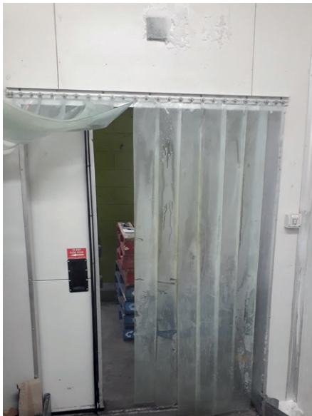
8 & 9. Strips hooked out of the way by staff leaving no thermal barrier
