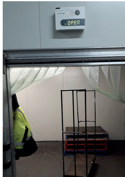
8 & 9. Strips hooked out of the way by staff leaving no thermal barrier
